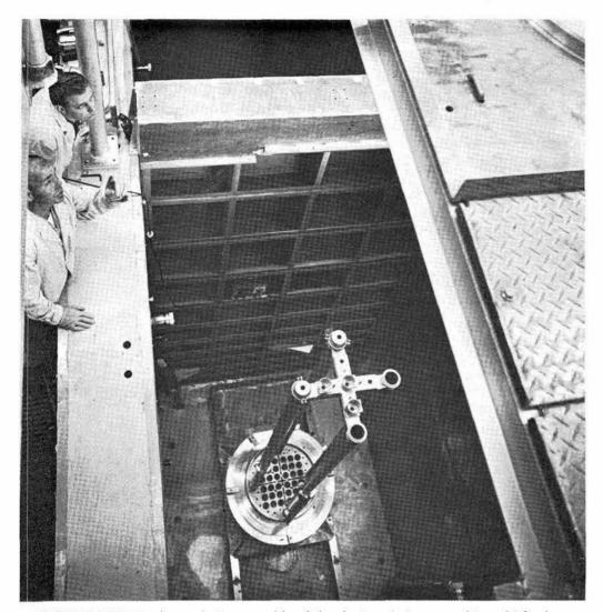
SNARE REACTOR is shown during assembly of the device. It is mounted in a 16-ft. deep pool of water with about 12 ft. of water covering the top of the core. Control rods extend about 10 ft. above the surface of the water. Control instrumentation is located on a balcony above the pool. At left are Roy Tackett of Reactor Division and Louis H. Sanders of Environmental Health Division.
